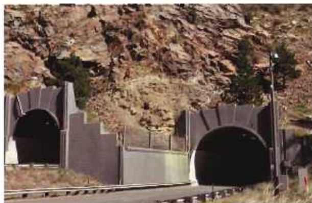
Figure 4. Original portals and original excavation.
