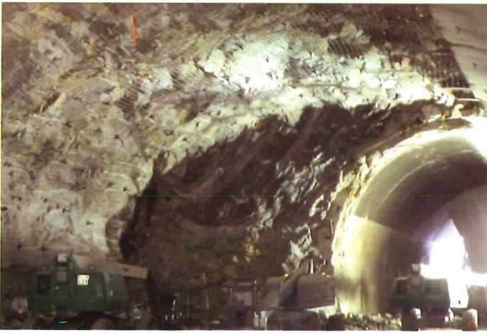
Figure 9. Tunnel blasted profile, drilled out blasting pattern.
