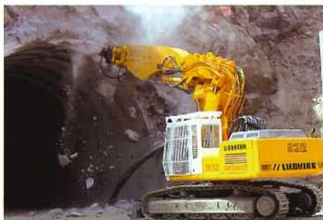
Figure 5. Saw cut operations and liner removal.
